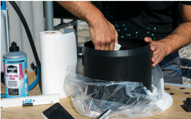
Clean the fusion zones of the fitting and pipe using Tangit PE-cleaner and a clean cloth.
