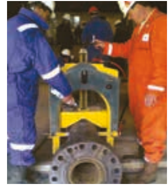
Guillotine cutting pipe
