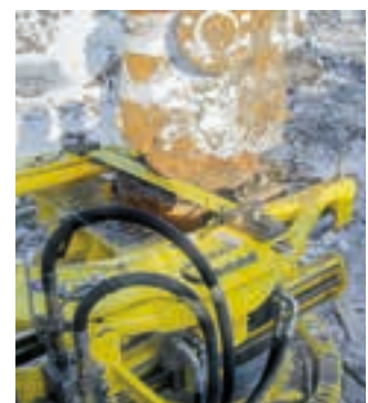
Guillotine cutting wellhead
