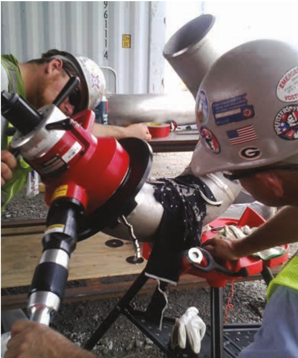
Box header beveling with SDB
