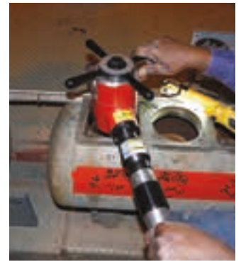
Box header beveling with SDB
