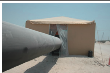
Protecting the welding zone using a tent
