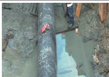
Water residues must be pumped off
